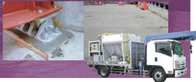
No shrinkage & high strength grout,
